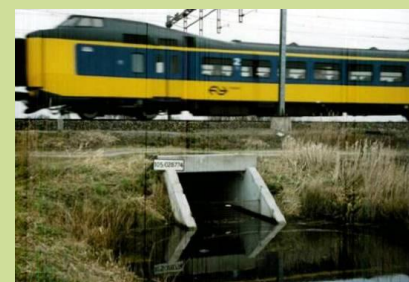
Fig. 1 – Passage on a culvert
